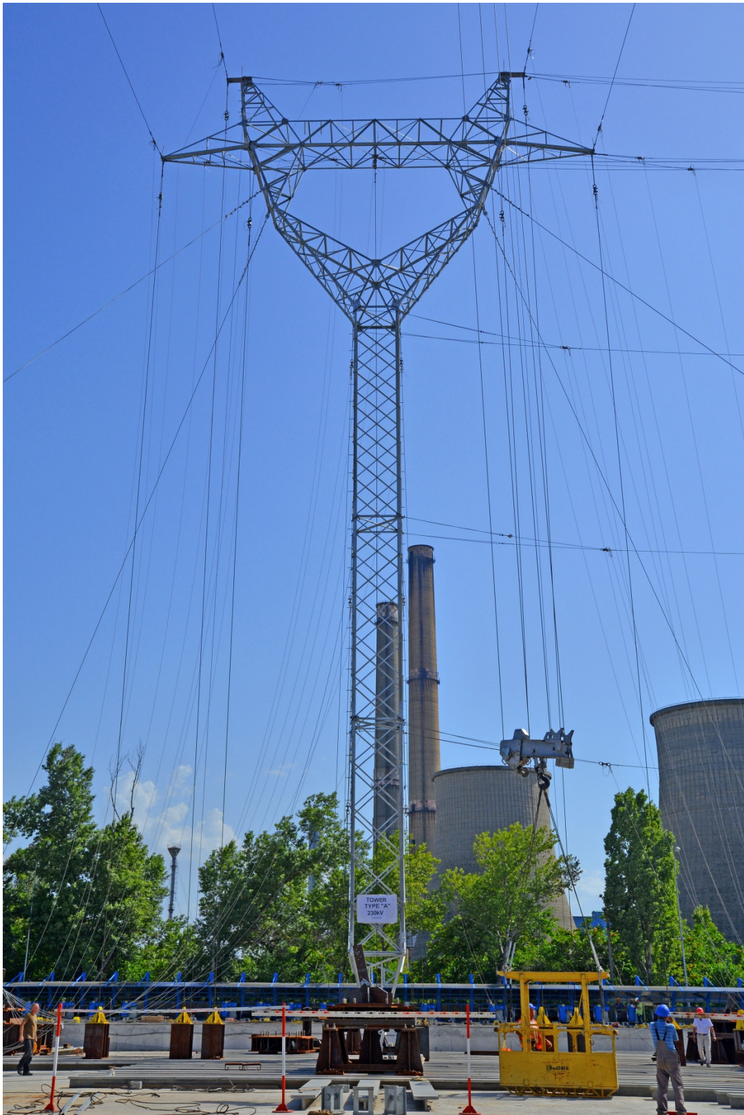
A-Tower Full Scale Load Test - Romania
