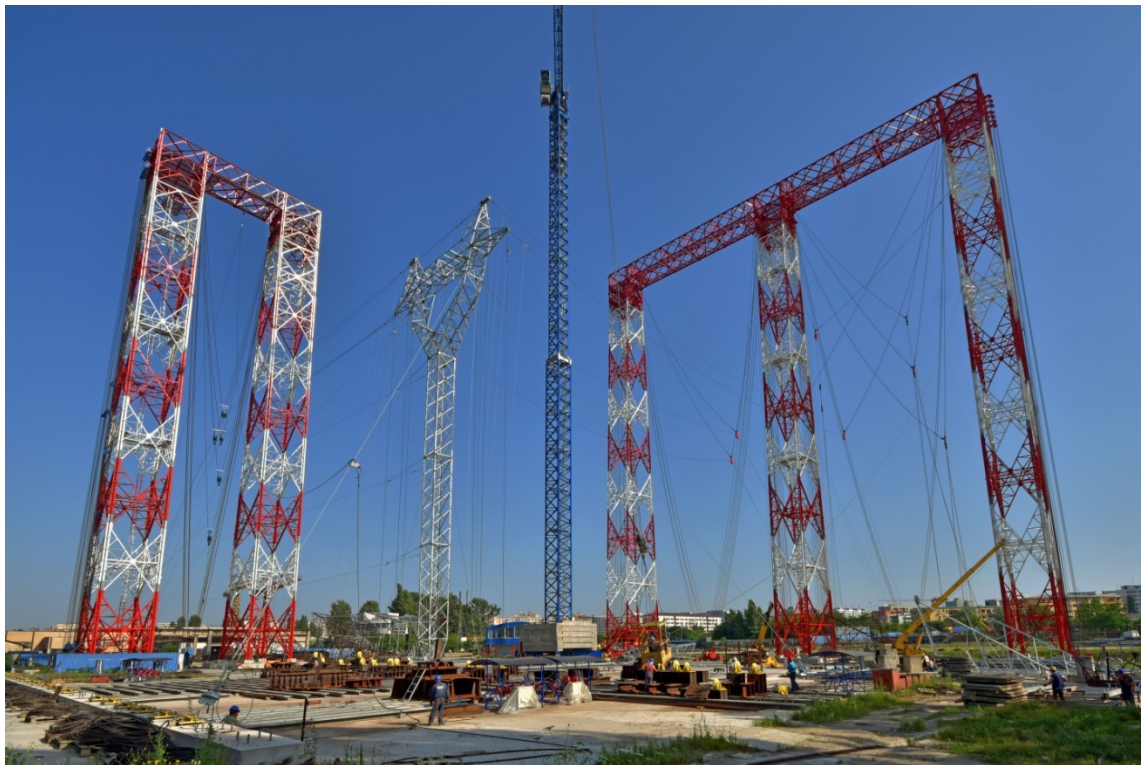
A-Tower Full Scale Load Test - Romania
