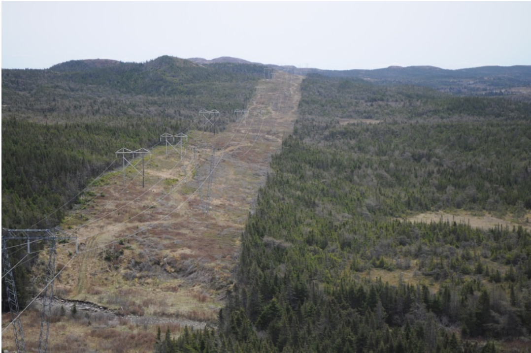
Typical TL203/TL237 right of way on the Avalon Peninsula; TL267 will be on the right
