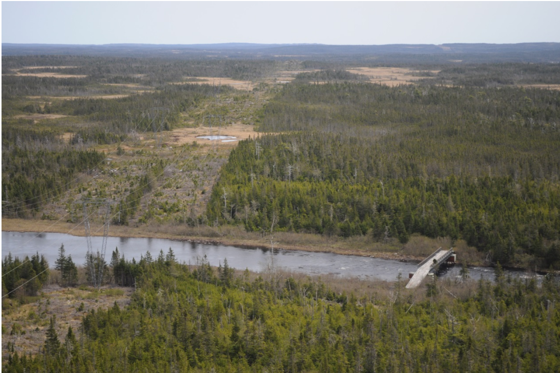
TL202/TL206 right of way with existing Hydro access bridge within the Bay Du Nord Wilderness Reserve
