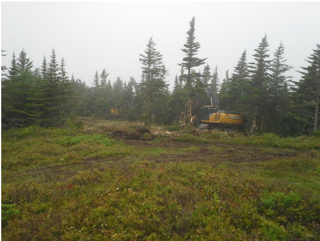
Start of Clearing Near Chapel Arm – June 27, 2016
